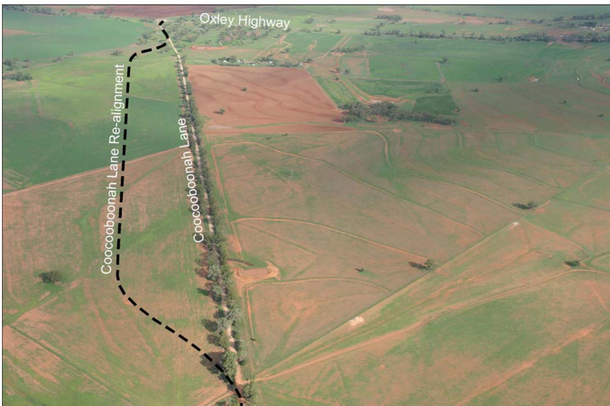
Plate 12 An oblique aerial view to the southeast along the proposed route of the Coochooboonah Lane re-alignment. Ref: E675B023
