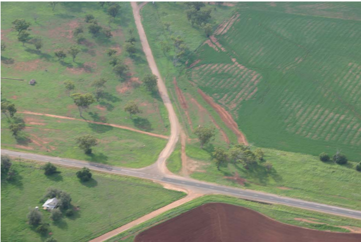
Plate 13 An oblique aerial view to the northwest across the existing intersection of Oxley Highway and Coocooboonah Lane. Ref: E675B-008.
