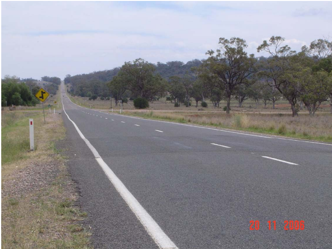
Plate 4 Oxley Highway Looking West at Coccoofoonah Lane Intersection
