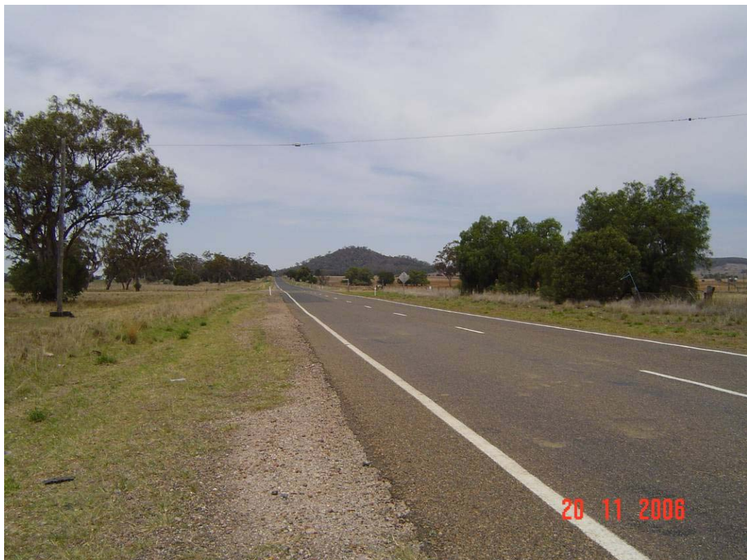
Plate 3 Oxley Highway Looking East at Coochooboonah Lane Intersection
