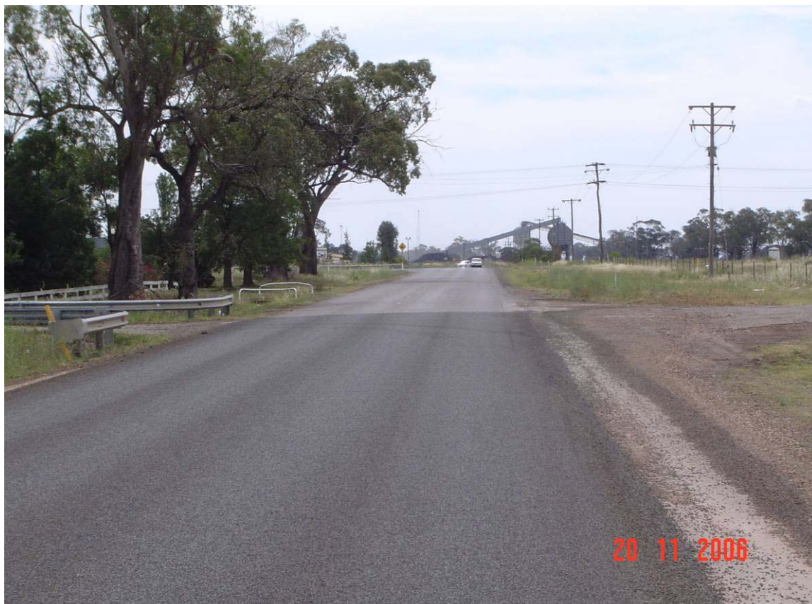
Plate 7 Quia Road Looking West at Blackjack Road Intersection
