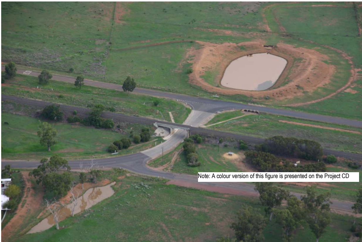
Plate 15 An oblique aerial view to the south across the rail underpass on Quia Road. Ref: E675B-001
